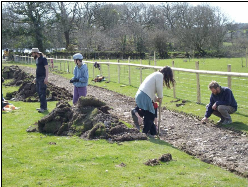
Renovating the trackway, March 2009
